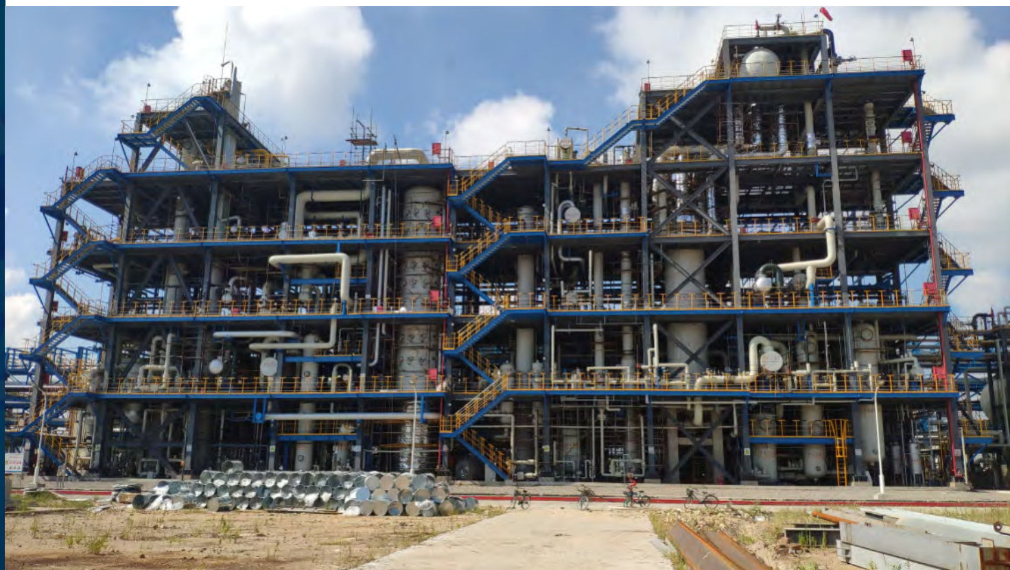
Figure1: 50 kt/a industrial facility for ethylene hydroformylation to produce propanal/n-propanol
