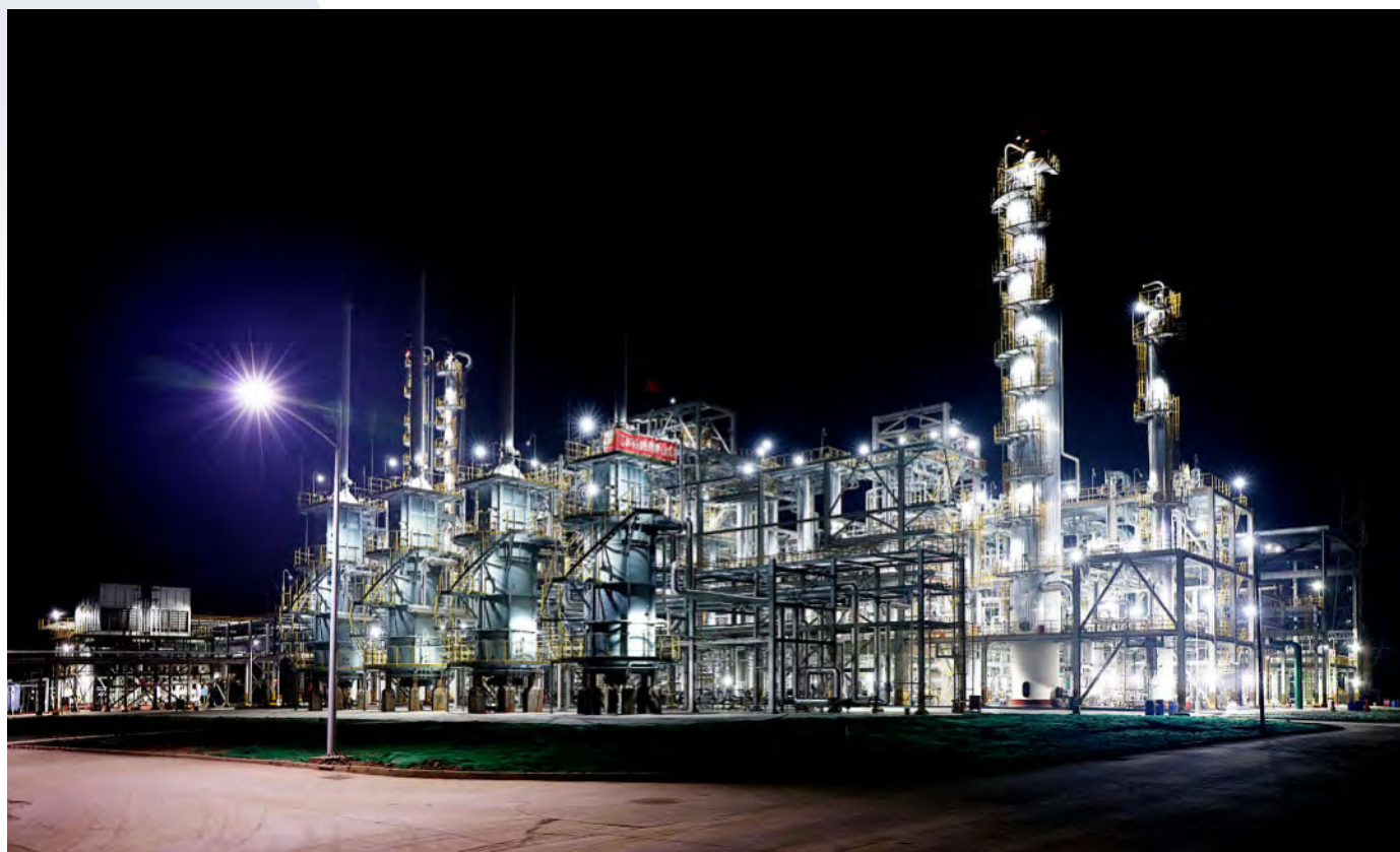
Figure1: The 100,000 t/a methanol to ethanol project
