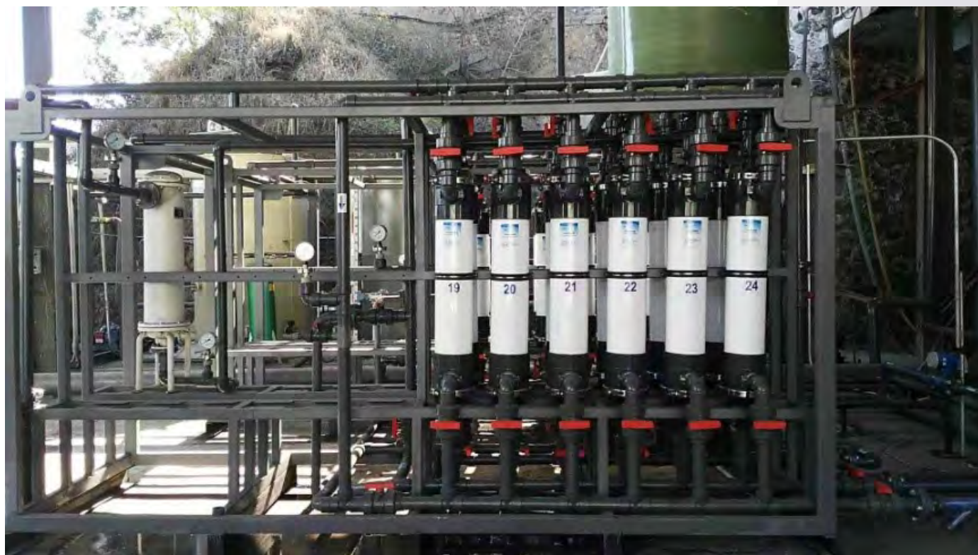
Figure 4: PTFE membrane contactor for the treatment of ammonia-nitrogen wastewater
