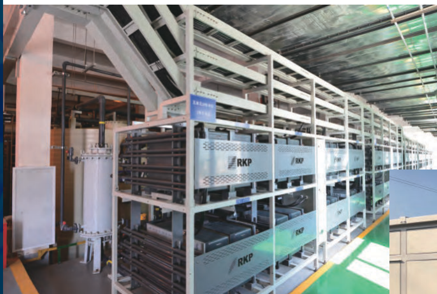
Figure1: 5 MW/10 MWh vanadium flow battery demonstration system
