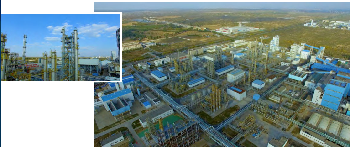
Figure 1: The 100 kt/a industrial demonstration plant for higher alcohol synthesis from syngas
