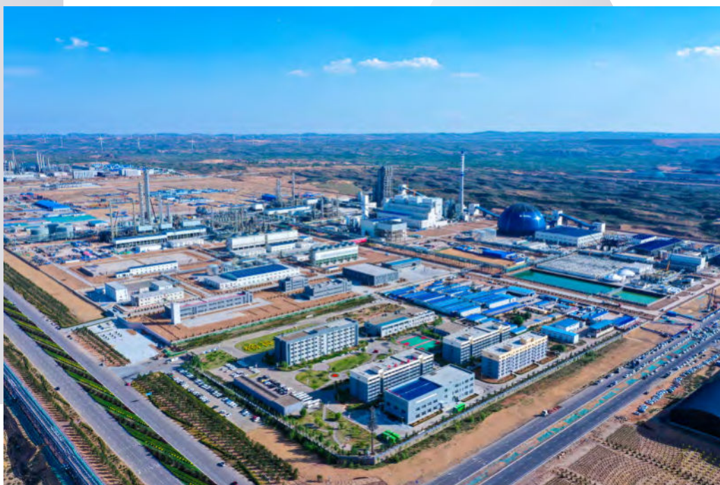
Figure3: 500 000 t/a methanol to ethanol plant under construction
